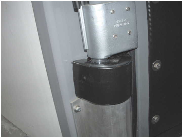
The Solid Riser snaps onto the Hinge Post above the Pillow Block and Over the top of the Lower Hinge Guard
