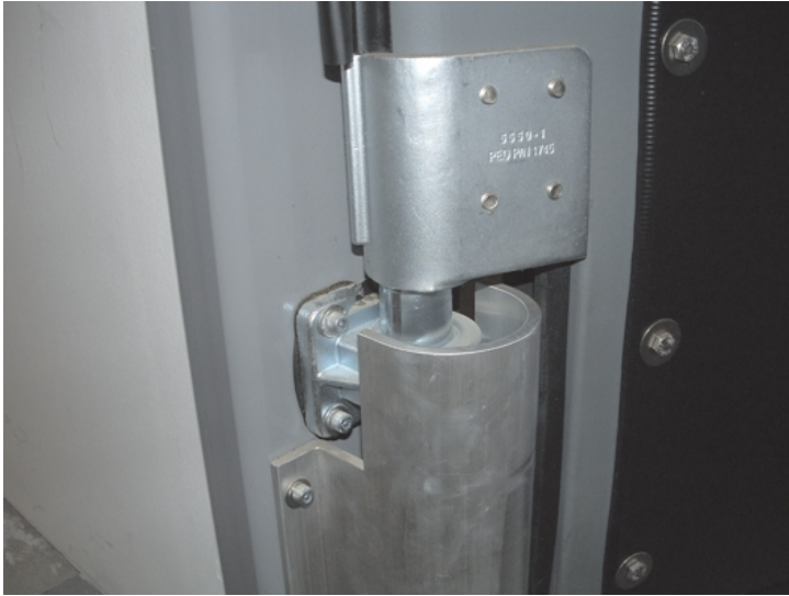
Door and Hinge Assembly must be completely installed prior to installing the Solid Riser
