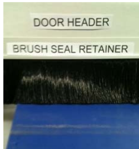
View looking up at door header
