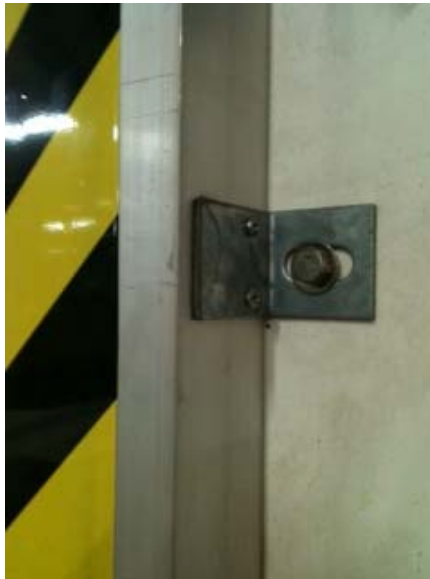
Guide Track Mounting Bracket
