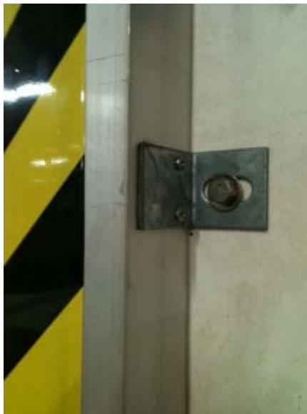
Guide Track Mounting Bracket
