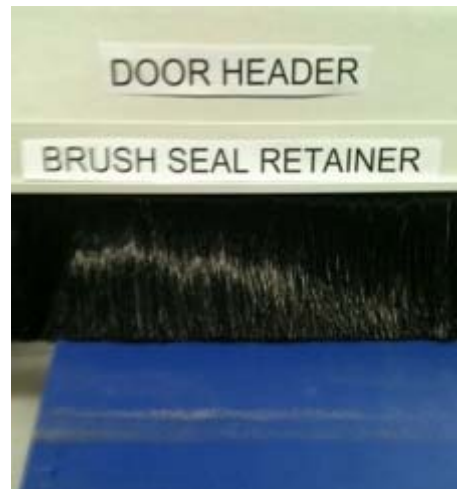
View looking up at door header
