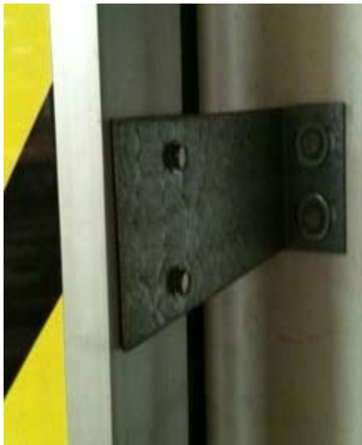
Extended Guide Track Mounting Bracket
