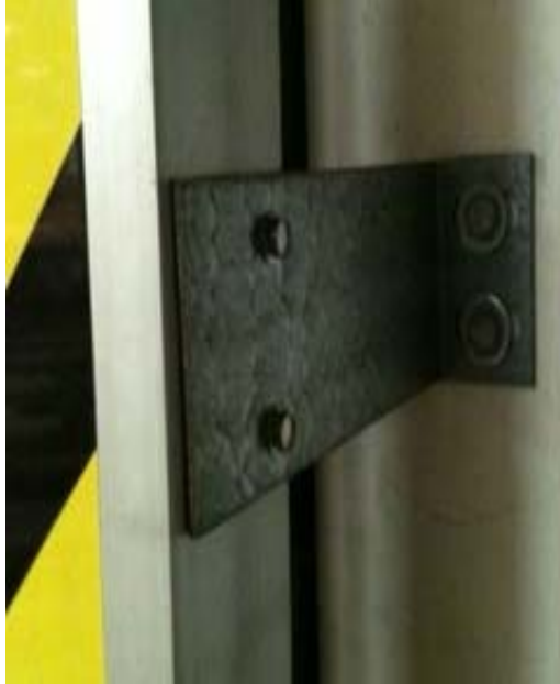
Extended Guide Track Mounting Bracket
