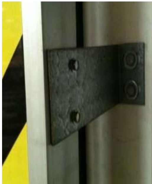
Extended Guide Track Mounting Bracket
