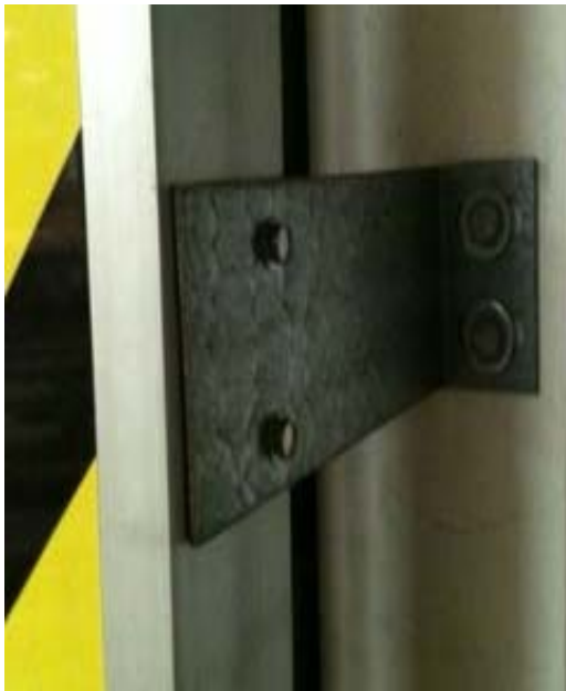
Extended Guide Track Mounting Bracket
