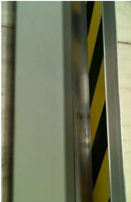
Guide Track Mounting Inside of door jamb
