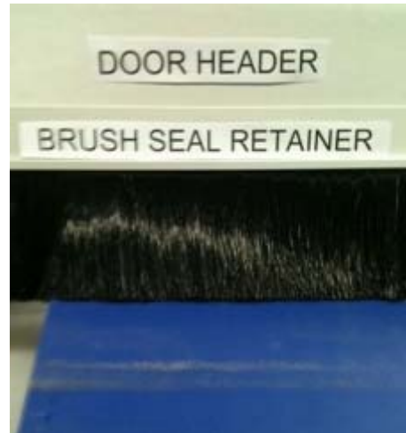
View looking up at door header
