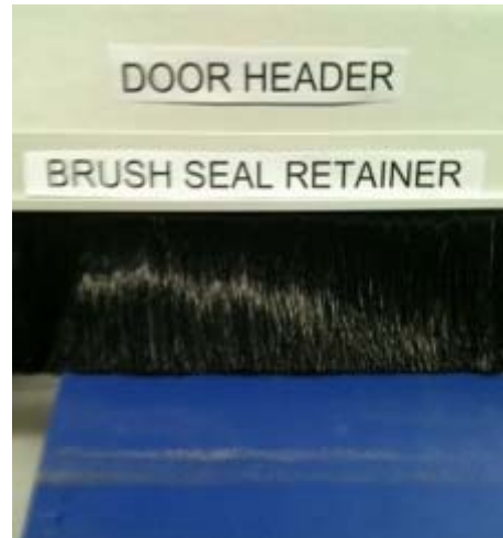
View looking up at door header
