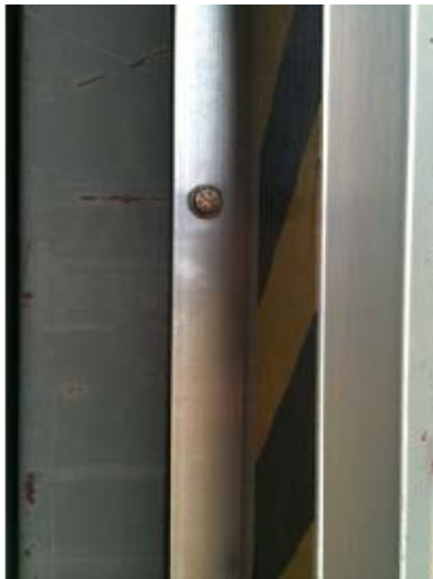
Guide Track Mounting Inside of door jamb
