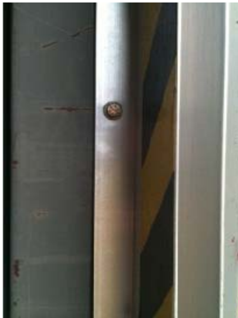
Guide Track Mounting Inside of door jamb
