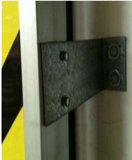
Extended Guide Track Mounting Bracket
