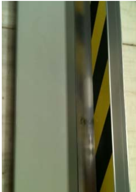
Guide Track Mounting Inside of door jamb
